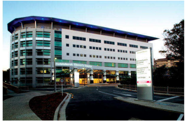
Part of Christchurch hospital
